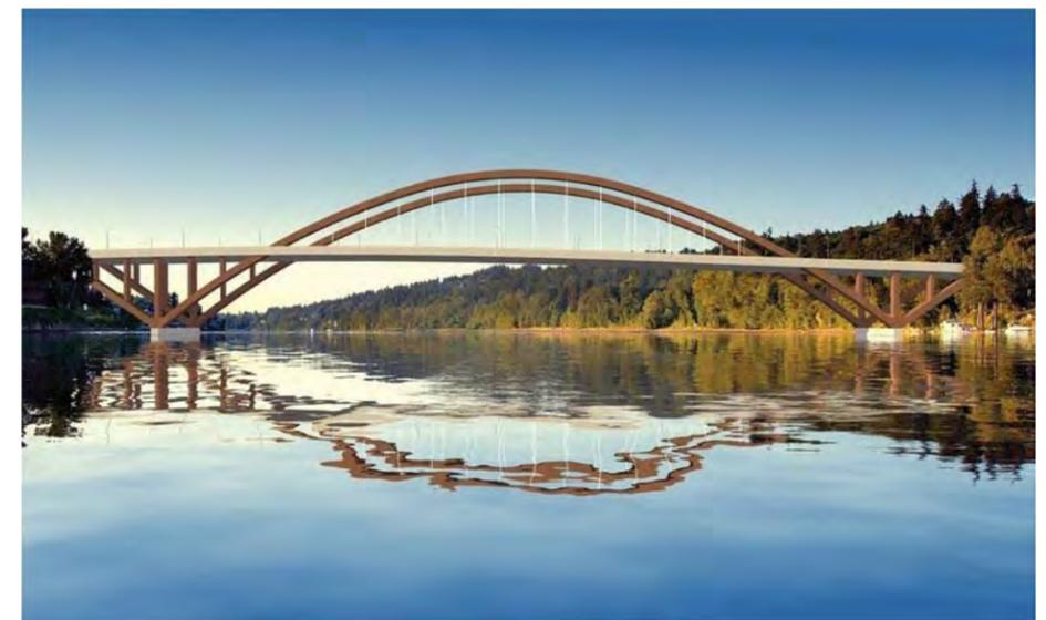
Example: A through-arch bridge with a lower return-arch
